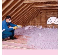
The AttiCat<sup>®</sup> Expanding Blown-in Insulation Machine conditions the AttiCat<sup>®</sup> Expanding Blown-in PINK FIBERGLAS<sup>™</sup> Insulation by breaking it up and fluffing it.
