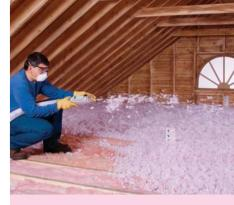
The AttiCat® Expanding Blown-in Insulation Machine conditions the AttiCat® Expanding Blown-in PINK FIBERGLAS™ Insulation by breaking it up and fluffing it.
